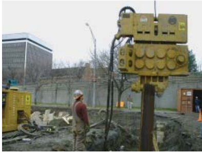
250VM with a sheet clamp driving sheets.
